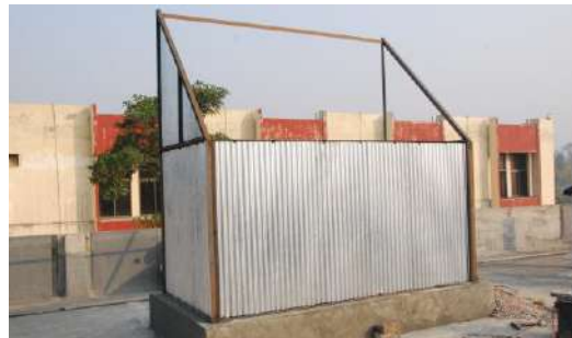
Hybrid Solar Dryer (Under construction) under ALP project # 001
