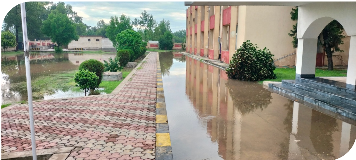
Damages due to heavy rain on August 8, 2024
