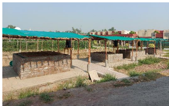
Zero Energy Cooling Chambers (ZECC) constructed at NIFA
