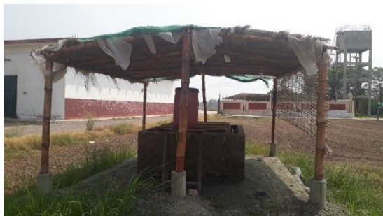
Zero Energy Cooling Chamber
